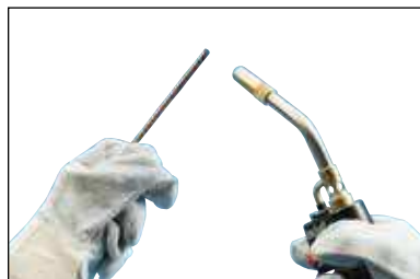
Fig. 4 The conductors should be clean and dry before the connection is made. Use a propane torch to dry wire conductors and remove remaining cleaning residue, solvent, or water before making the Cadweld One Shot connection.
