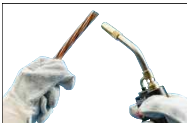
Fig. 11 The conductors should be clean and dry before the connection is made. Use a propane torch to dry wire conductors and remove remaining cleaning residue, solvent, or water before making the Cadweld connection.
