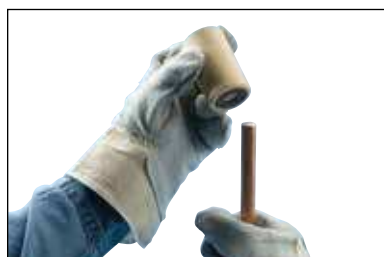
Fig. 6 Each Cadweld One Shot contains a rubber grommet at the bottom of the mold. Gently turn the Cadweld One Shot onto the ground rod until the ground rod reaches the stopper and cannot go any further.
