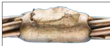
Fig. 29 Completed Cadweld connection.
