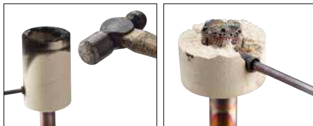
Fig. 15 Break the ceramic Cadweld One Shot mold off of the connection. Avoid contact with hot materials. See the “nVent ERICO Cadweld Quality Standards” section to see whether a quality connection has been made.
