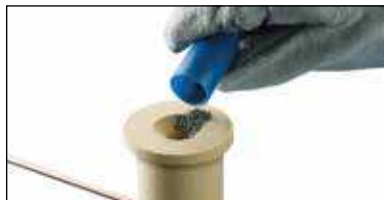
Fig. 14 Pour the starting material onto the Cadweld One Shot cover. NOTE: Welding material is an exothermic mixture and reacts to produce hot molten material with temperatures in excess of 2500 degrees Fahrenheit (1400 degrees Celsius) and a localized release of smoke. Avoid direct eye contact with "flash" of light from ignition of starting material. Avoid inhalation of smoke/fumes.
