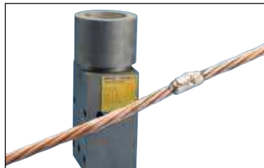
Fig. 31 Ready to make another Cadweld connection.
