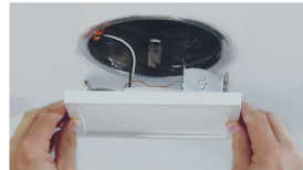
Friction clips for recessed housings
