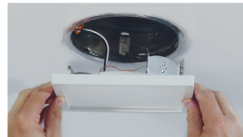
Friction clips for recessed housings
