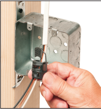
Feed cable into connector.
