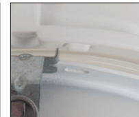
Align post on LED light module with the slot on the trim and place light module onto trim.
