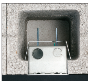
Insert the box in the opening in the block. (Top view shown)
