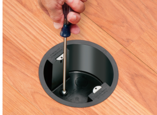
2 Secure box by tightening two #10 screws inside box.
