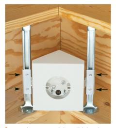
2 Loosen the screws noted above. Slide box along brackets to center it between rafters. Tighten screws. Install wires.
