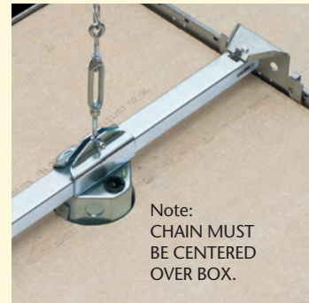
3 Use the "S" hooks provided to attach chain to turnbuckle, and chain to the overhead support. Use turnbuckle to apply tension to the chain, so it supports the weight of fan.
