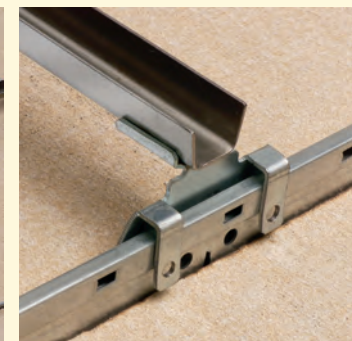
3 Snap ends of support bar over the ceiling grid (tees).
