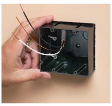
2 Pull wire through installed NM cable connector. Insert ONE-BOX.
