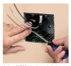
3 Mount ONE-BOX directly to stud with shipped in place screws.
