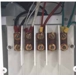
Copper Busbar with Ratings from 250 to 500 A
