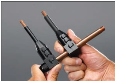
4. Slide connector/insulator assemblies onto rod.
