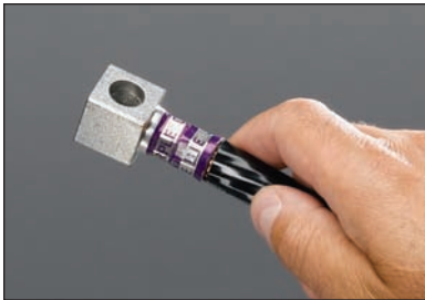
1. Crimp Multi-Tap connectors onto cables.
