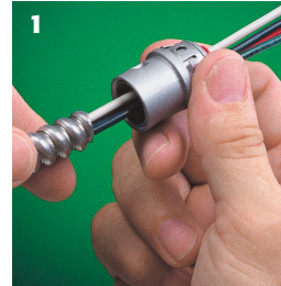
1 Snap fitting onto cable... twist clockwise
