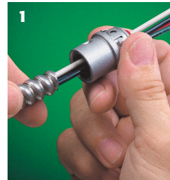
1 Snap fitting onto cable... twist clockwise
