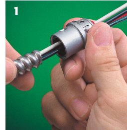
1 Snap fitting onto cable... twist clockwise
