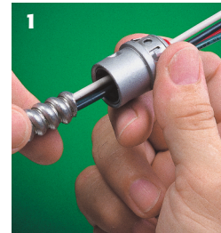
Snap fitting onto cable... twist clockwise
