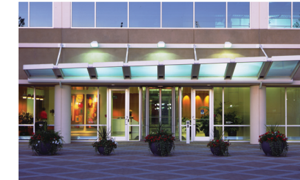
outdoor facility lighting
