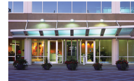
outdoor facility lighting
