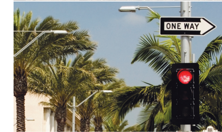
traffic signal controls
