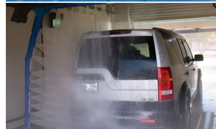
car wash controls
