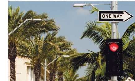
traffic signal controls
