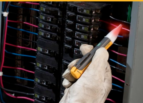
1AC-II with beeper, on-off and self test
